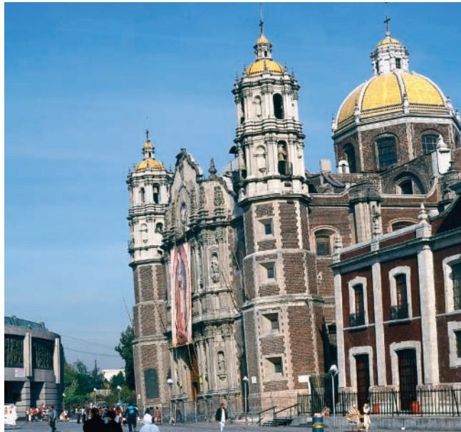
FIGURE 13.29 Subsidence of buildings in Mexico City resulted from compaction after groundwater was pumped from unconsolidated sediment beneath the city. Subsidence has caused this building to tilt and sink more than 2 m.
