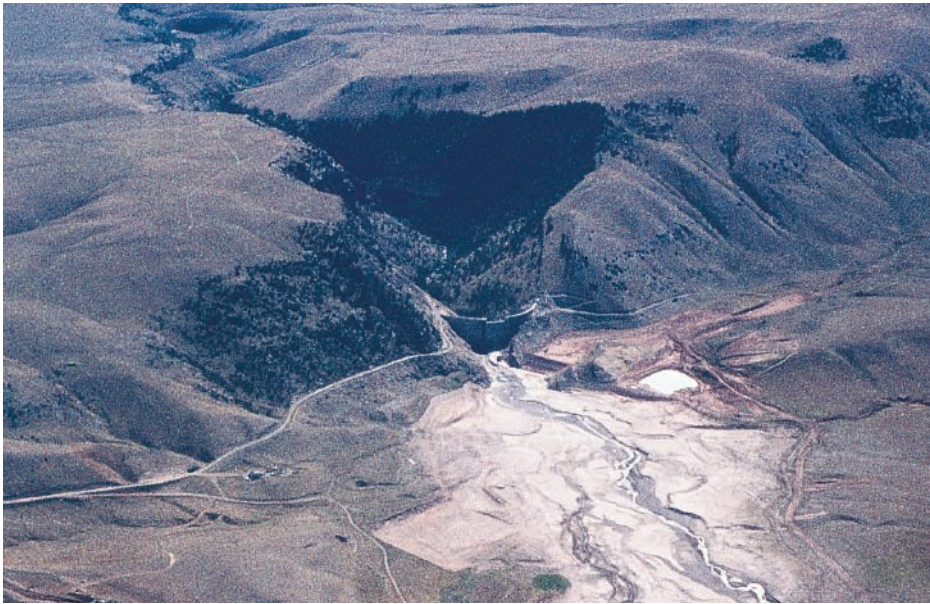
FIGURE 13.30 A dam constructed on permeable limestone in western Wyoming never functioned because the surface water seeped into the subsurface. The dam lies at the beginning of the gorge. The light-colored sediment behind the dam marks the fraction of the reservoir that formed before water was lost through seepage.
